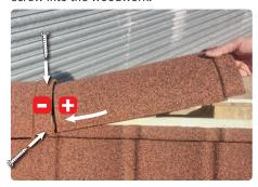
Continue adding the ridge tiles in the same way until the length is completed. The end cap fits onto the *male* end of the ridge tile, so you may need to make a spacer using another cut ridge tile.
