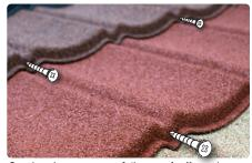
Overlap the next row of tiles **vertically** and screw through both tiles into the side of the batten. Continue laying rows to the apex of the roof.
