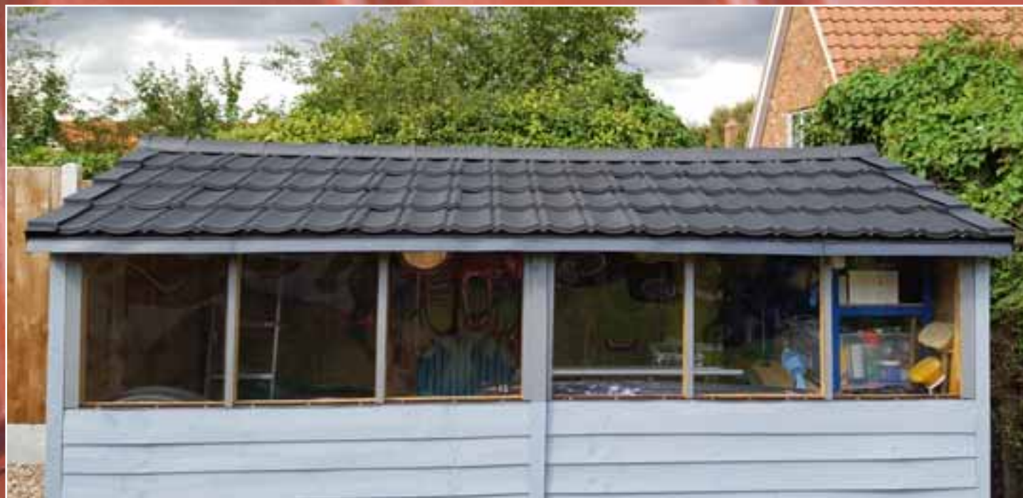
BEFORE FITTING SMOOTH TILES
