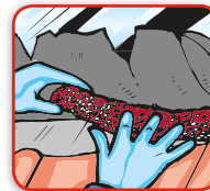
Repairing torn lead flashing
