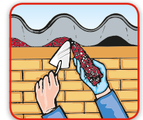
Sealing of corrugated roofs
