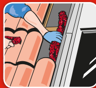
Adhering tiles to roof windows
